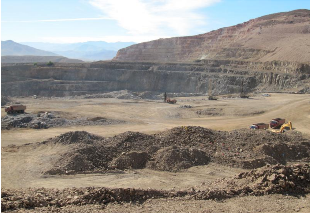
Figure 4 –Blast Hole Drilling at Churrumata (background) and mining Mariposa Vein (foreground)
