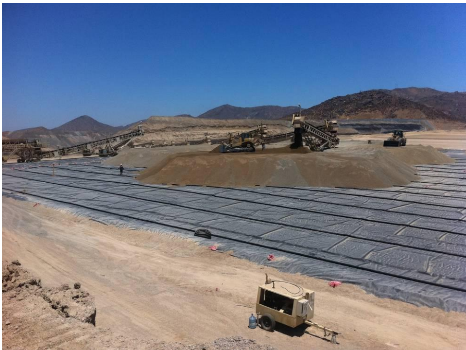
Figure 1 – Ore being stacked on pad 3 b
